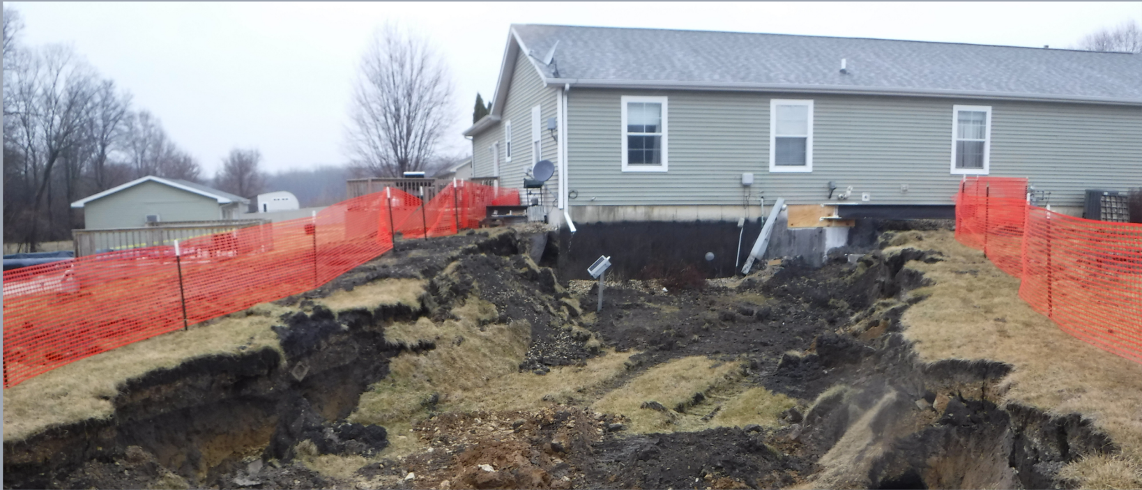
Example of Pit Subsidence - Limestone Mine
