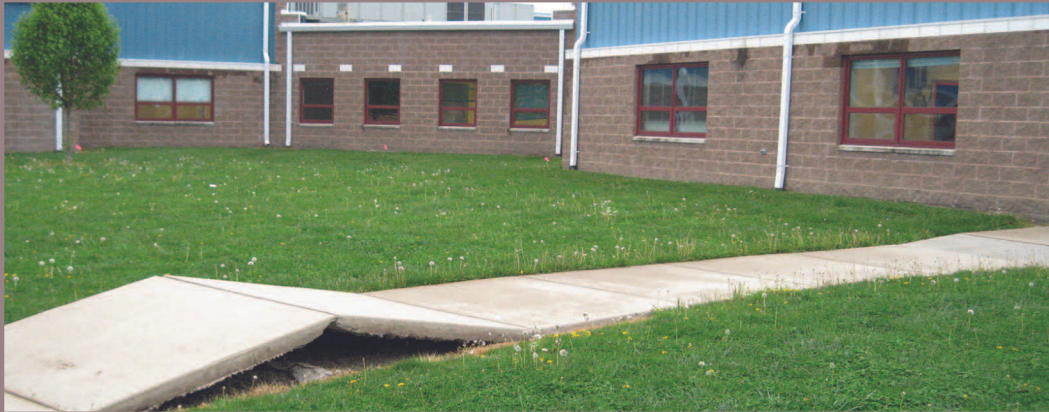
Example of damages from Sag Subsidence
