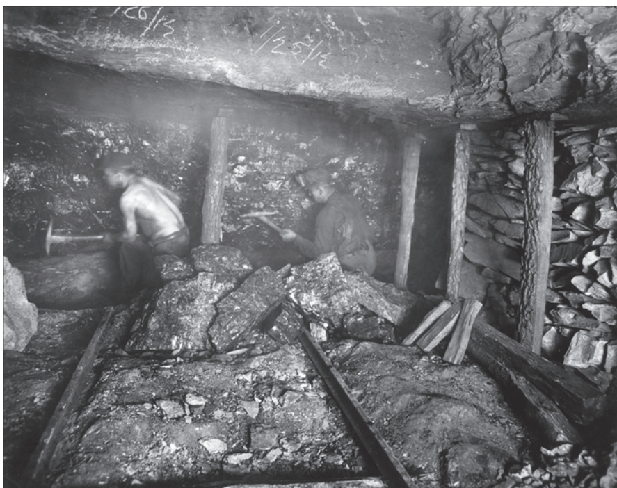
Figure 5 Photograph of mining at the face in an early longwall mine. Note the stacked rock support on the right side. More than 145 of these mines operated from 1856 to 1954 in 18 counties. Most were located in the northern counties from Bureau, LaSalle, Grundy, and Will (fig. 2).
